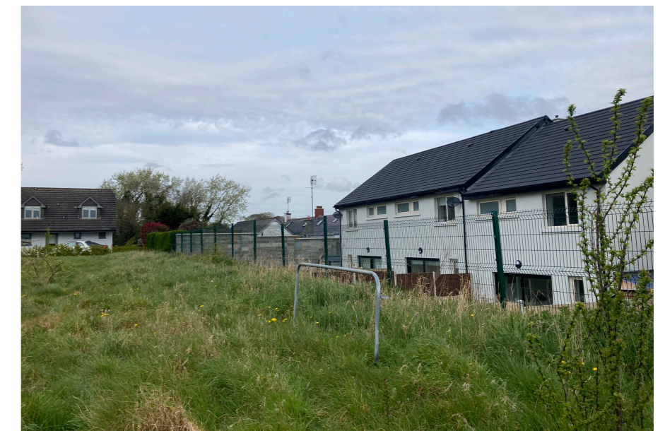
Figure 3.16: Existing boundary in northwest corner (paladin fence on a retaining wall). The proposed development will provide for privacy with a concrete post & timber panel fence inside this boundary
