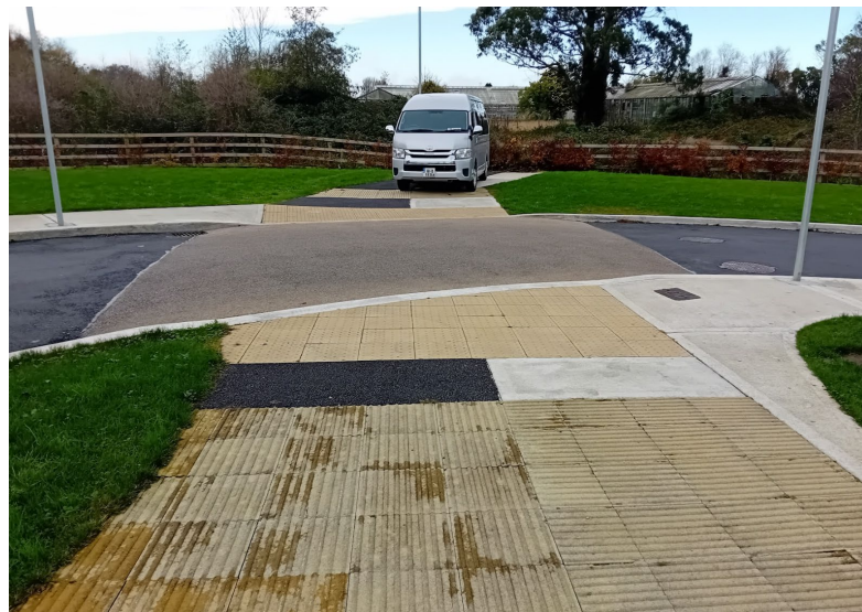
Figure 7.2 – Tie in to existing footway and pedestrian infrastructure
