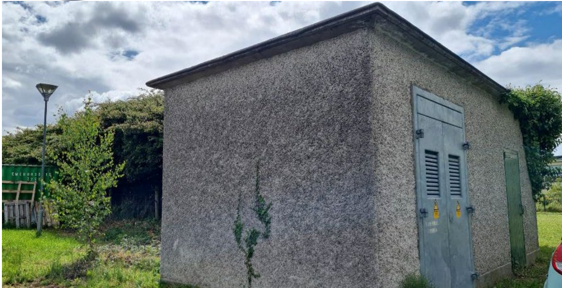
Building 12 at former offices
