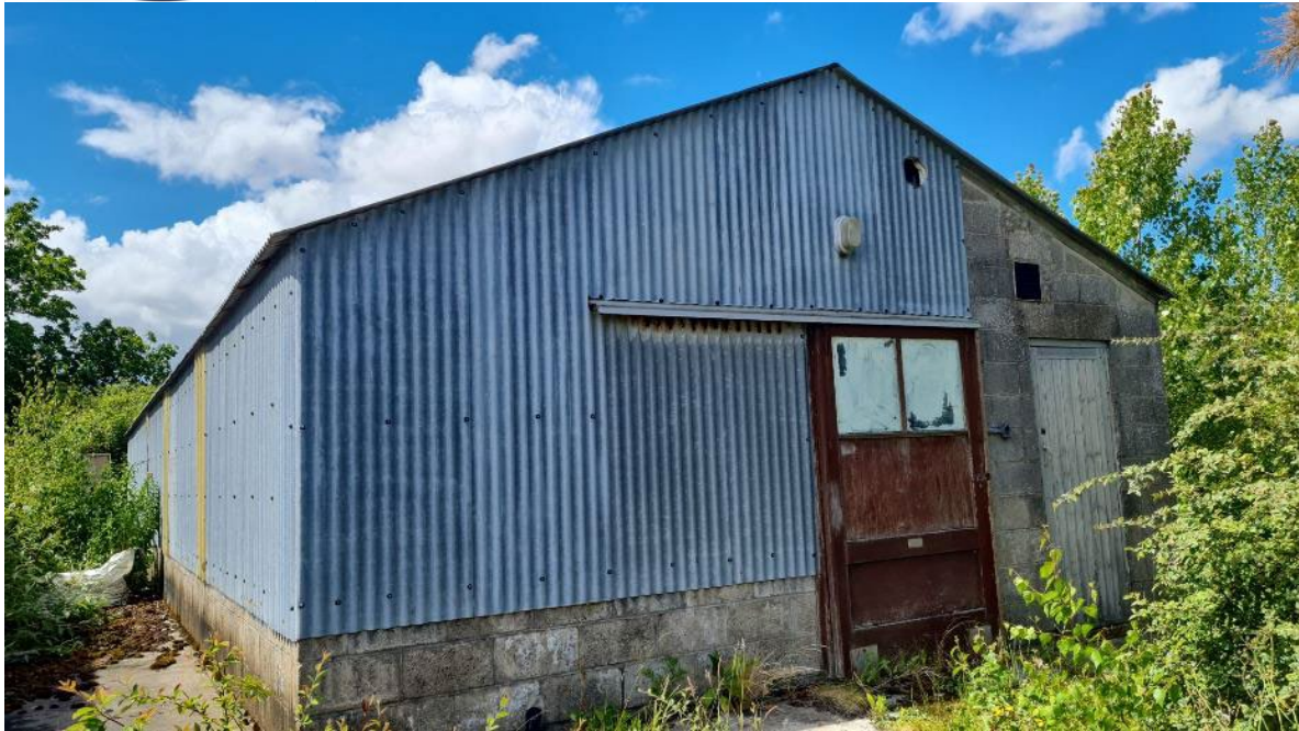
Building 5 – Northern shed
