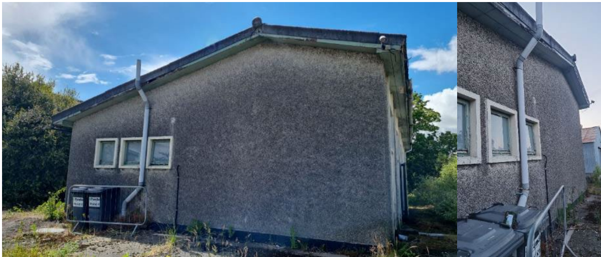
Building 4 – Large shed and Mini location June 2024
