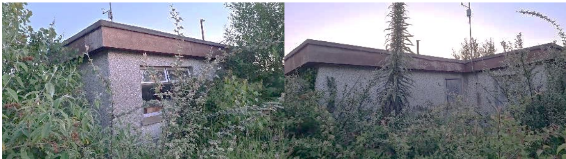
Building 11 – Storage building on perimeter
