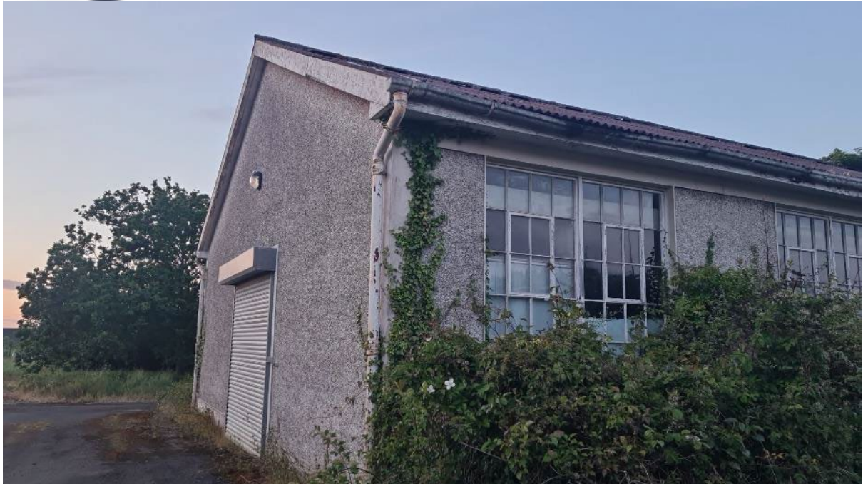
Building 3 – Stores and location of Mini September 2023
