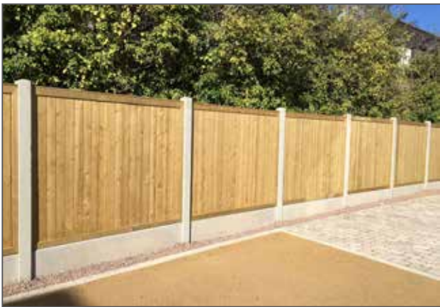
Residential Boundary Fence Timber Panel & Concrete Post Fence w/ gravel board 1.8m high
